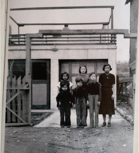
Original Eng Family Backyard Gateway - New design will be larger scale to accommodate hanging a larger gate
