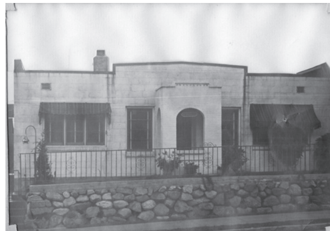
Ca. 1940 with the addition of the concrete curb and decorative railing, and enclosed porch
